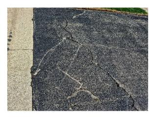
For what ever reason, either the initial build quality was less than satisfactory, or the fact that they are in shade throughout the winter – resulting in a deeper frost depth and increased frost *heave*, these driveways have not lasted as long and are now deteriorating. This was pointed out by the engineer conducting the on-site Reserve Fund Study Property Inspection.
